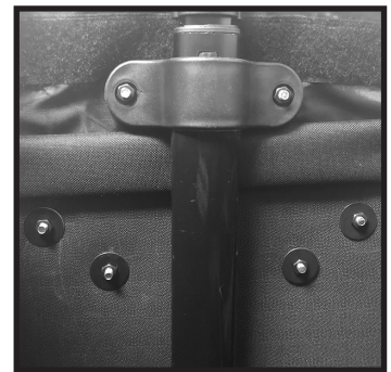
Pic #8 - Finished Interior
