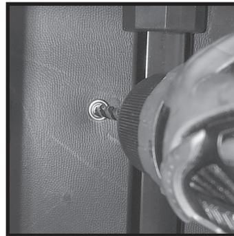
*Pic #3 - Drill out rivet*
